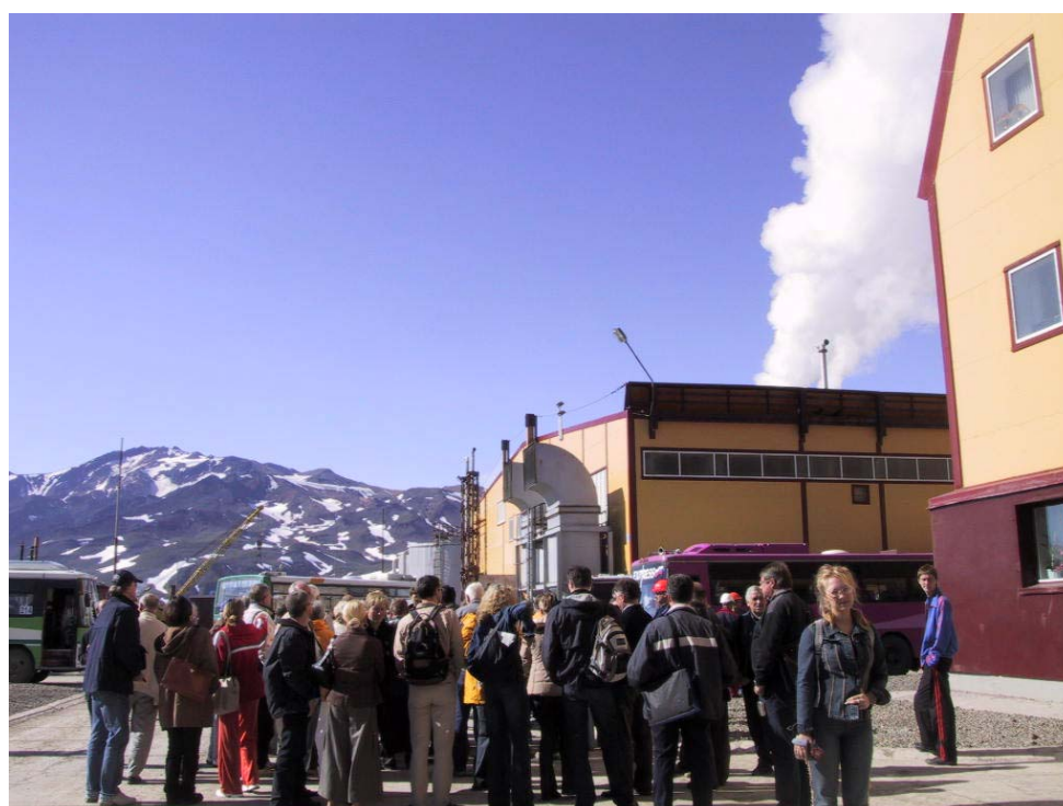
Figure 4,a. Mutnovsky geothermal power plant. Many visitors always. Photo of Svalova V.B.
